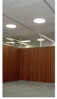
RIGHT: In the basement, the meeting rooms are illuminated by sunlight DEPLO-SUN GLASSTOP lines, offering lots of light to these spaces for your particular distribution does not have windows. The result is a connection to the outside through the natural light provided by the ducts.
