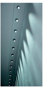
LEFT: Parans fibraóptica modules are installed on the roof of the building, where capture and concentrate sunlight and transported by fiber optic cables into the interior. This system illuminates the press room and the stairs of the building lobbies. Sunlight comes through swiveling terminal bathing the walls and creating pleasant lighting effect or natural. If a cloud passes, light fluctuations, just as would happen with a skylight.
